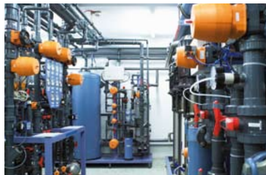
As a contractor, REMONDIS Aqua extended the facilities owned by WILD Valencia S.A and then took over the operation of them. The wastewater treatment process is now used to generate biogas which, in turn, is used to generate steam for the production processes.
