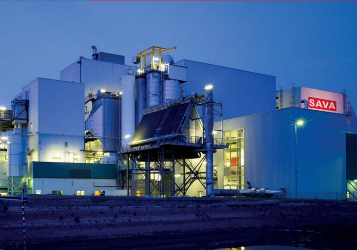
Hazardous waste must be disposed of correctly to prevent unnecessary environmental pollution
